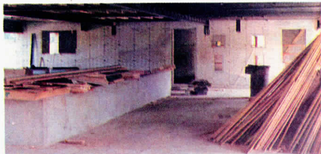
Once completed, big bales will drop through floor of big bale storage loft into concrete feeders below.
